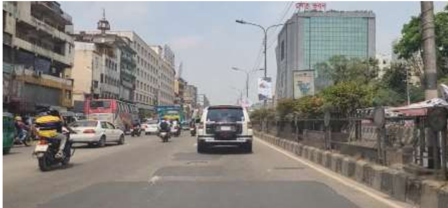
Figure 19: Pothole after flyover before Shainik Club
