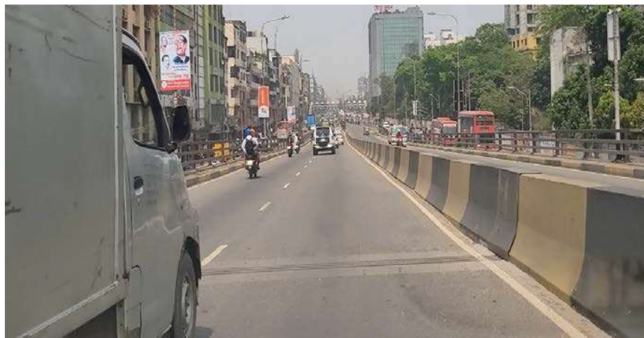
Figure 18: Expansion joints at Mohakhali flyover
